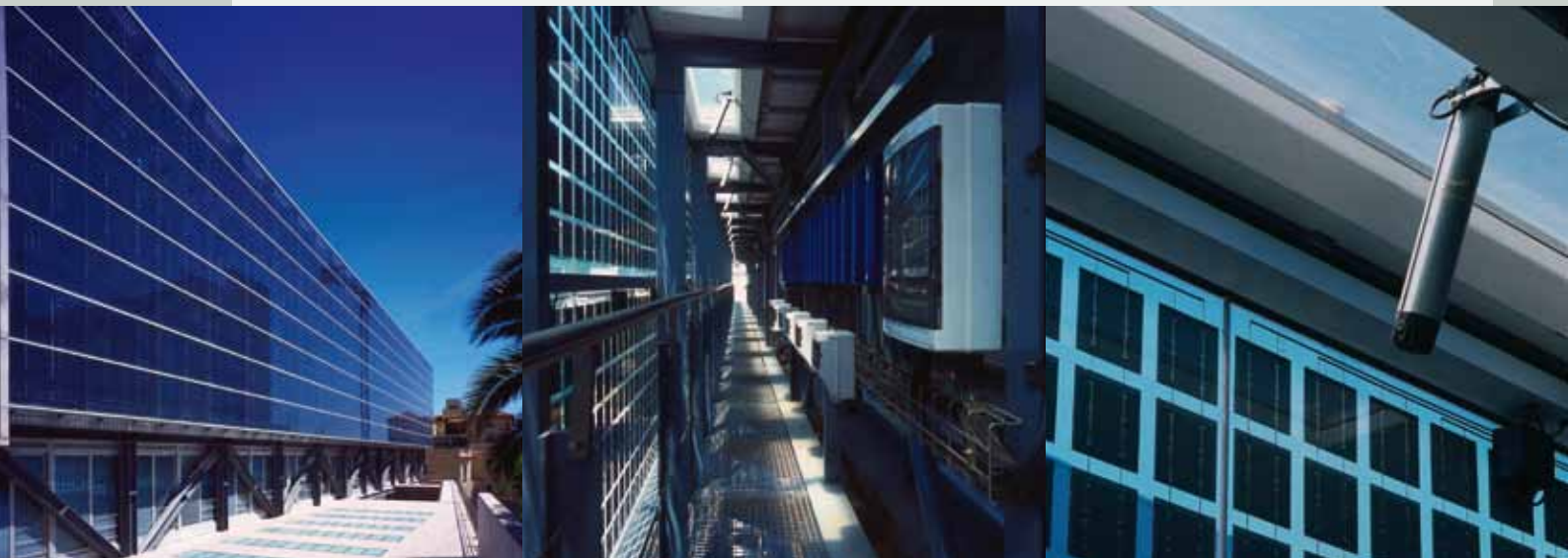
Curtain wall with photovoltaic panels - La Salle - Barcelona, Spain (Architect : Robert y Esteve Terradas Muntaniola)
